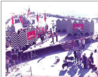
Figure 2.4 For this 1967 ABC prime-time entertainment show, Operation Entertainment , the deck of an aircraft carrier served as an outdoor studio. To eliminate any potential problems with cable slack as the tide rose, the production truck was hoisted onto the deck. Notice the camera stage right. It was a second-generation color camera, a PE-250 from GE. It was equipped with a 10:1 zoom lens, standard at the time. Camera heads used to be much larger than their lenses; now the opposite is true. (Source: Jerry Hughes)
